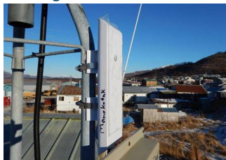
NanoStation receives Network Service or Wireless Internet Service from GCI the Alaska statewide Cell provider, excellent GCI system
